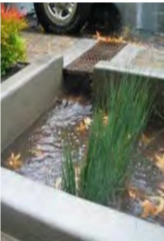
Filtering water in a contained curbside retention area.
